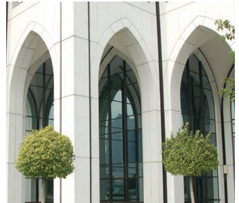
Gothic Arch Lintel
