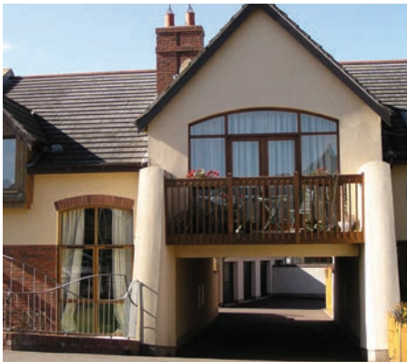
Segmental Arch Lintel
