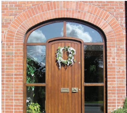
Parabolic Arch Lintel
